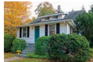
421 Roses Mill Rd, Milford $264,000
