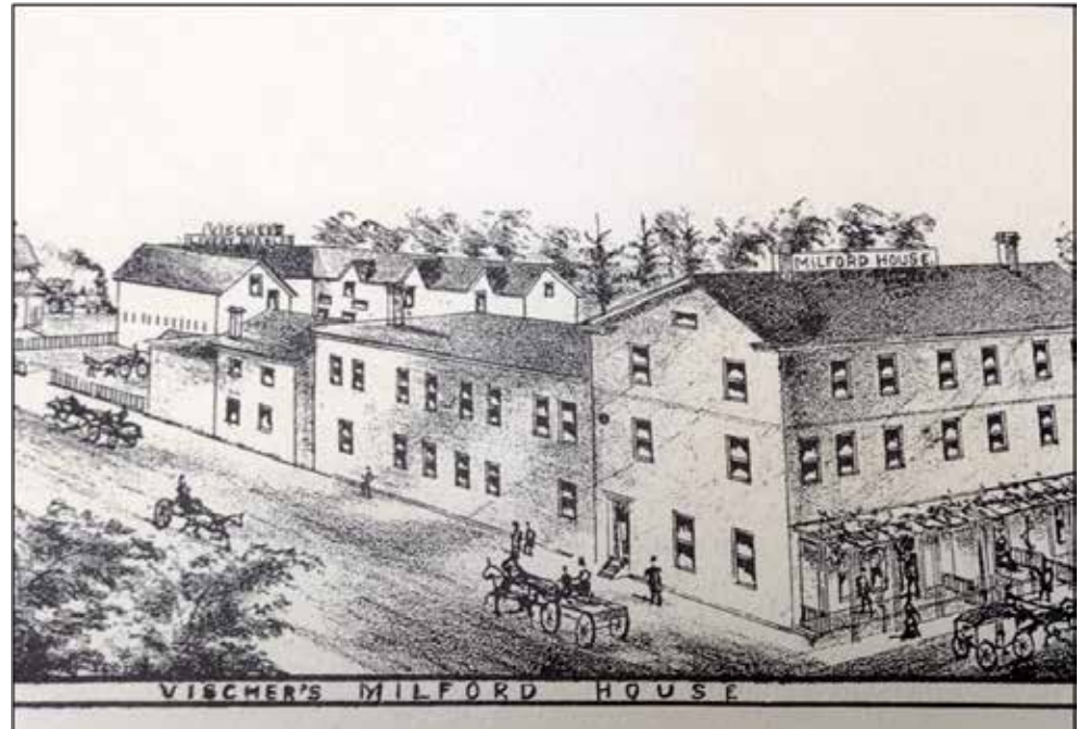
This drawing of the Milford House and Vischer’s Stables is from an 1882 engraving by the O.H. Bailey & Co. of Boston. Oakley Hoopes Bailey (1843–1947) was known for producing panoramic, bird’s-eye views. The eastbound railway station is at the far left of this picture. Photo courtesy of the Daniel E. Moger photo collection.
