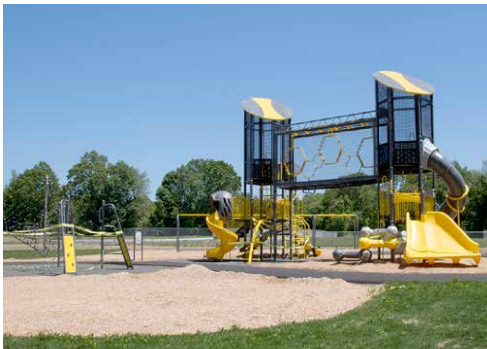
The community playground at Fred Wolfe Park in Orange is nearing completion, with the main playscape elements fully installed. It will be Orange's first public playground not attached to a school. Photo by Lexi Crocco.
