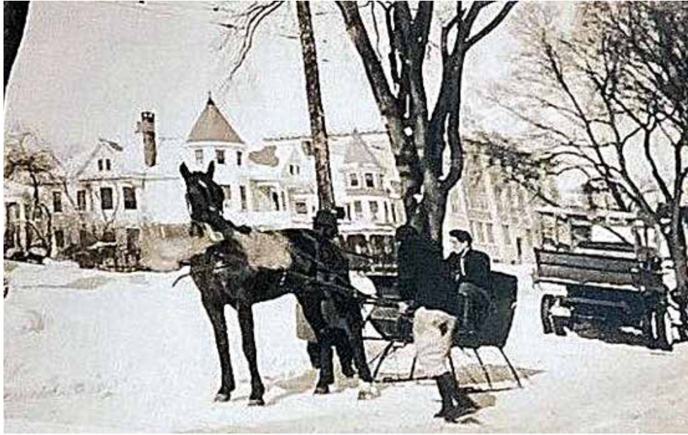
This handsome horse looks like he's ready to take off for a wonderful winter sleigh ride after a heavy snowfall in the 1930s. Notice the beautiful houses in the background. They were all destroyed. The only structure still standing is the Diane S. Toulson Building that in 1986-1987 narrowly escaped destruction. Today that building is the River Park Apartments for seniors on West River Street.
