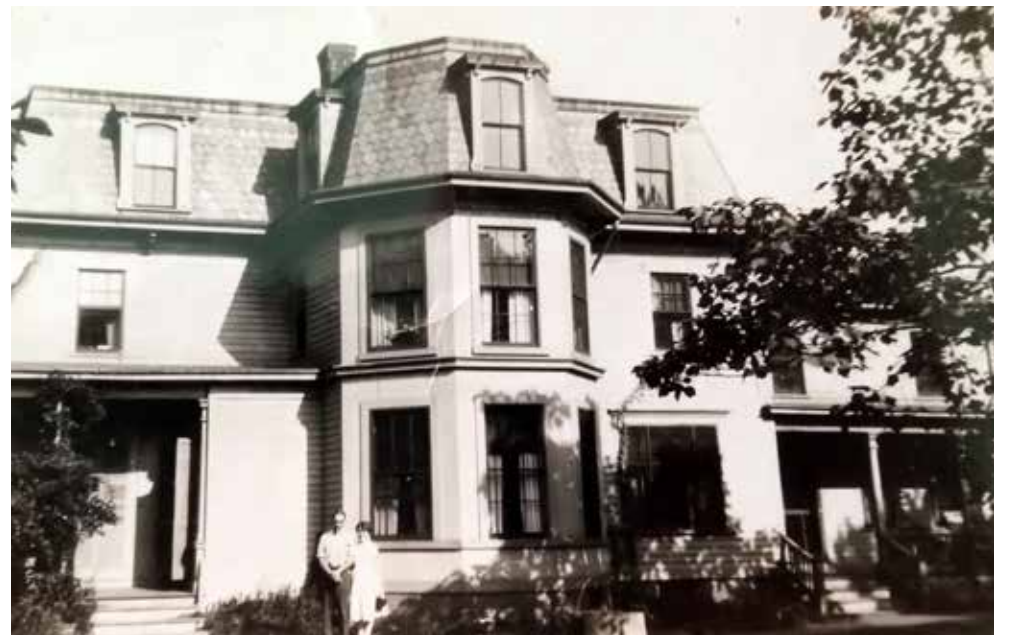
The Dumraese residence. Franz and Ida Dumraese are in front. Photo courtesy of Paul Dumraese.
