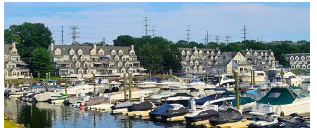
The Caswell Cove condominiums are situated next to the Housatonic Wastewater Treatment Facility in Milford. Photo by Brandon T. Bisceglia.
